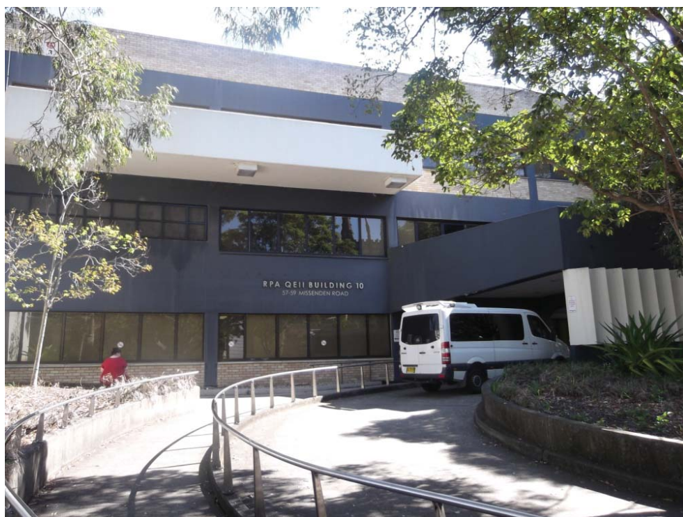
Figure 10 RPA building at 57 Missenden Road
