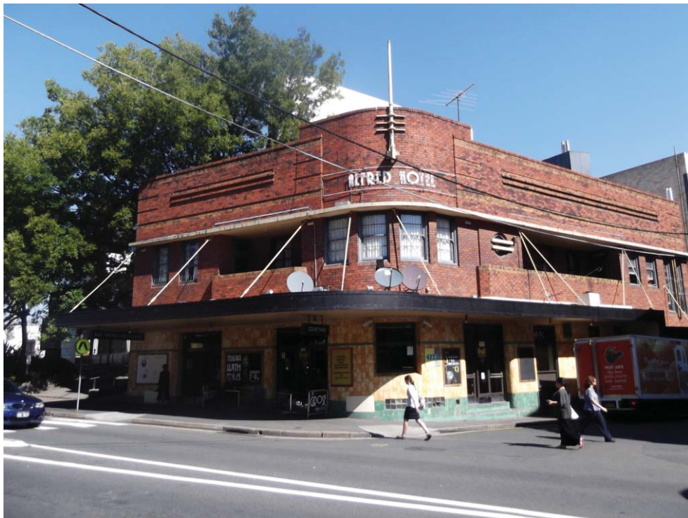
Figure 3 View from Missenden Road
