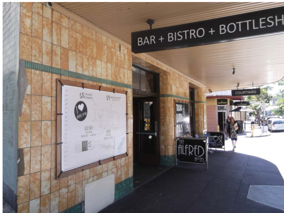
Figure 5 Front entry on Missenden Road
