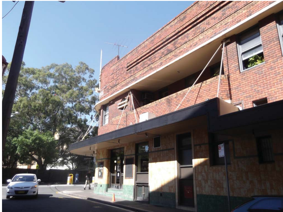
Figure 4 View from Dunblane Street
